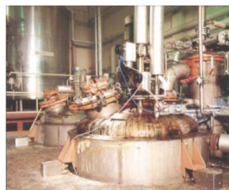
Batching Process Reactors and Process Vessels
